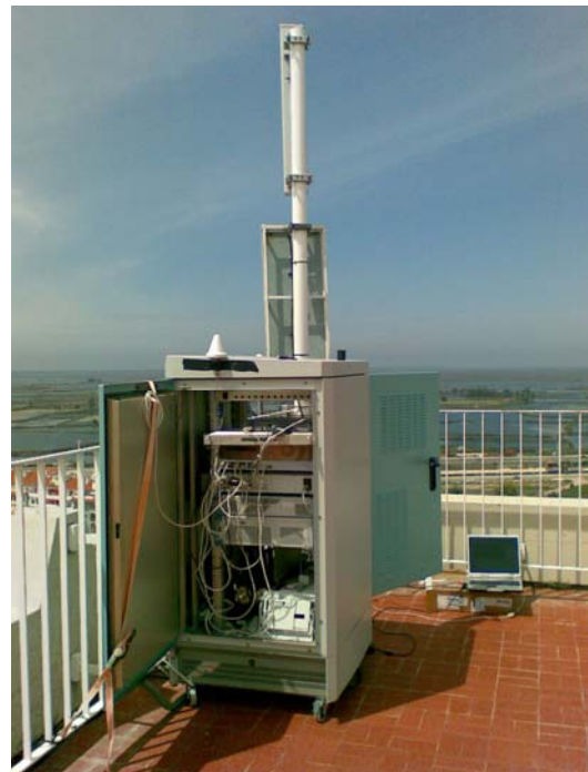
Fig. 2. SUIT transmitter in a shelter. WiMAX 2.5 GHz antenna is on the top of the mast.
